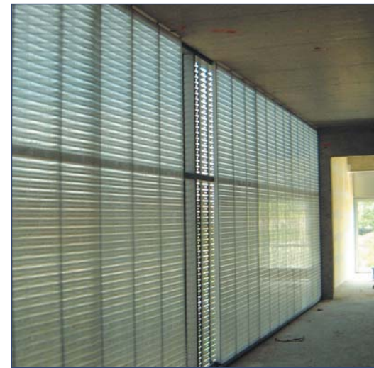
Danpalon and perforated metal cladding create a striking effect
